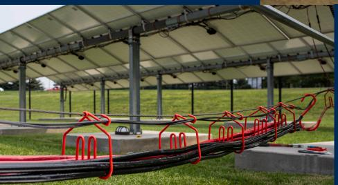
Choose CAB<sup>®</sup> Solar for tracker, ballasted or fixed installations. CAB<sup>®</sup> multi-carrier hangers safely separate bundles of cables to meet NEC requirements. Numerous standard designs are offered to safely support large bundles of string wires, DC feeders, as well as AC, data or other cabling. Ask about custom hanger configurations to meet specific project requirements.
